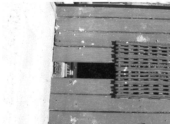
This missing decking board is a safety hazard and needs to be rectified immediately.
