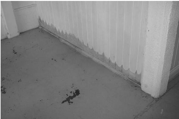
This wall was water damaged. An improvement in both waterproofing and surface drainage was required to rectify the problem.
