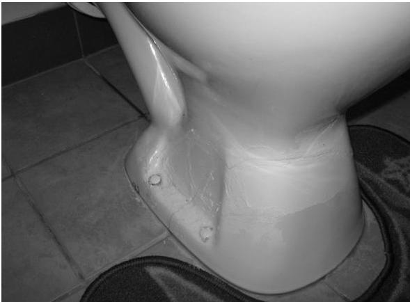
This cracked toilet pan should be replaced before it collapses
