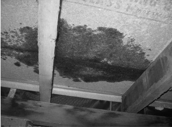
This stain under a particle board floor is damage from a water leak. Further investigation by a licensed plumber is recommended. If the leak is not promptly repaired the flooring may have to be replaced in this area.
