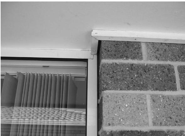
This gap was around 8mm wide at the top of the wall. There were other gaps and cracks also present in the house, so the client was referred to a
