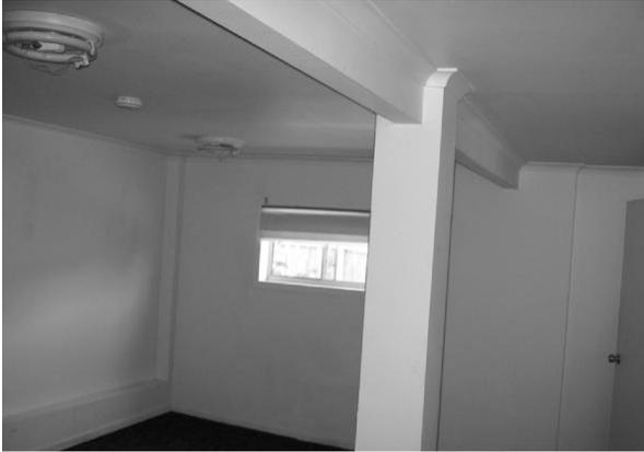
Here is a typical example of a room built under a house. The beam and post supports have been enclosed with plasterboard. The ceiling height in these areas should be checked with a tape measure.
