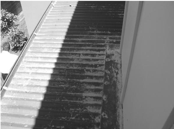
The renderer left this mess all over a brand new roof. The builder was not even aware of it. We found this defect during a handover inspection of a new house.
