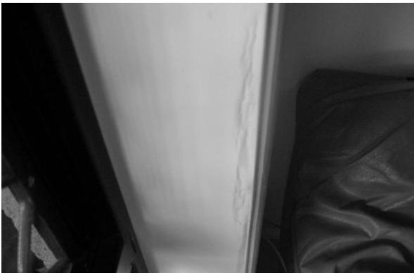
Suspected termite damage found to this internal timber required an invasive inspection.
