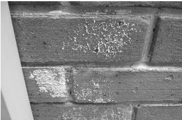
This is an example of efflorescence on brickwork.
