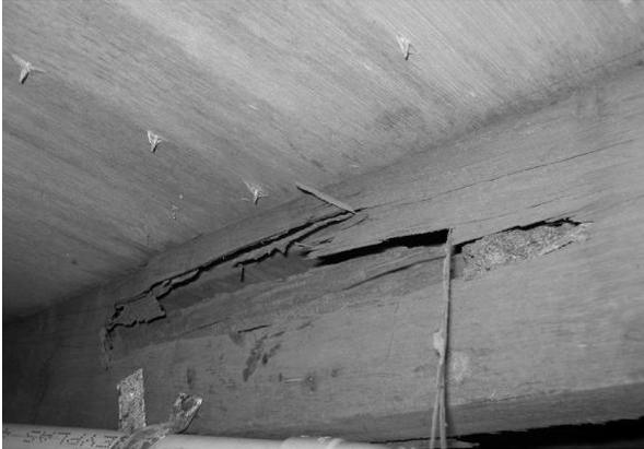
Subterranean termite damage to a hardwood floor joist. This joist had to be replaced.
