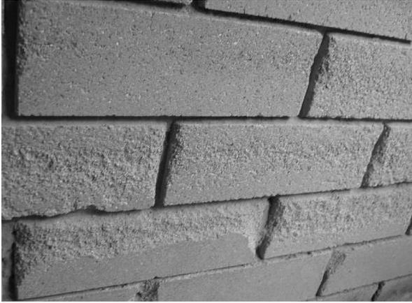
Crumbling bricks are known as fretting. Usually the damage is only minor and non-structural. Sometimes the damage is severe and extensive, and a lot of repair work is required. Refer this to your building inspector for assessment.
