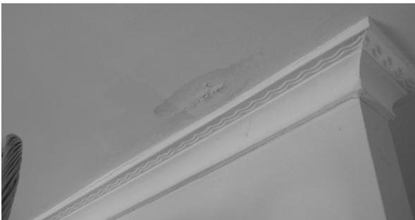
Your building inspector can check leak stains with a moisture meter.
