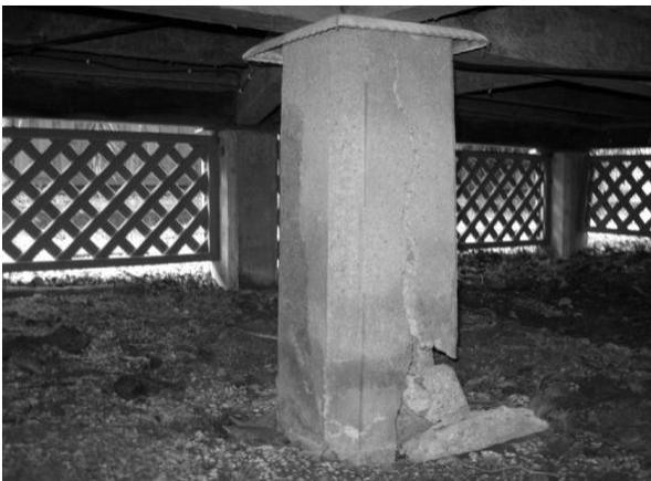
Concrete posts will often crack when the steel reinforcement inside the post is exposed to dampness. The steel rusts and expands, causing the concrete to crack. Cracked posts should be replaced.
