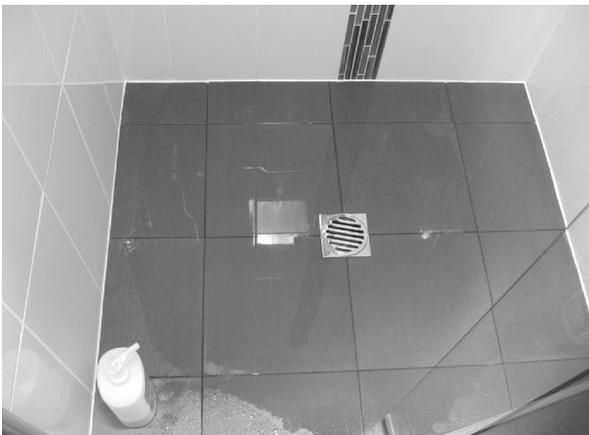
This shower base was installed with insufficient fall to the drain. It had to be rebuilt.
