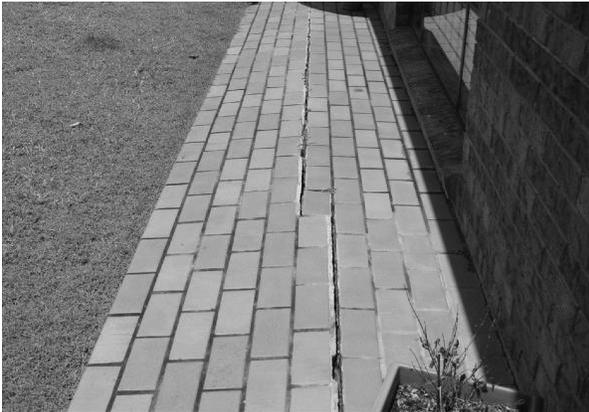
Cracked paths such as this one are a potential tripping hazard and should be replaced.
