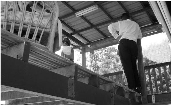
There is a balustrade missing on the edge of this deck. This is a safety hazard that needs immediate rectification.
