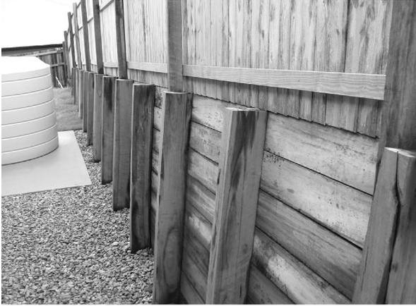
An example of a well-built timber retaining wall. All timber is H3 treated hardwood. Posts are 200mm x 100mm at 1.2m centres and sleepers are 200mm x 75mm. The wall has a slight batter (leans back towards the top).
