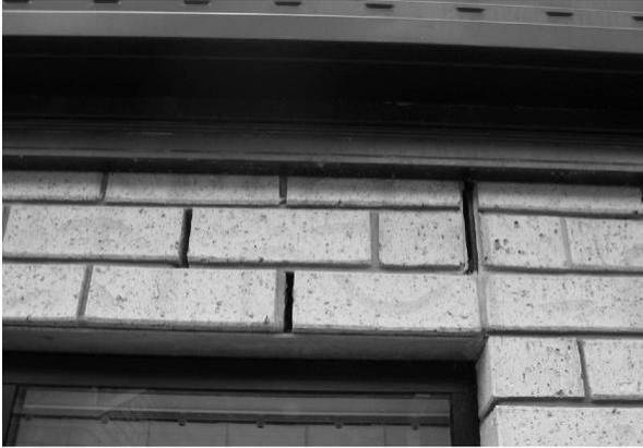
A structural engineer should be consulted about any significant cracks. The cracks in this photo are approximately 10mm wide.
