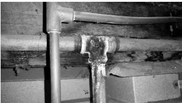
Rusting galvanised pipes are likely to also have rust in the inside. This can reduce water quality and pressure. Discuss the necessity of replacing
