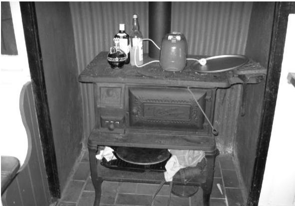
There was combustible material adjacent to this pot belly stove. This installation was unsafe and had to be rectified before being used again.
