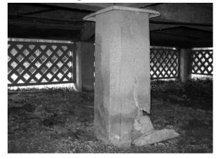
Concrete posts will often crack when the steel reinforcement inside the post is exposed to dampness. The steel rusts and expands, causing the concrete to crack. Cracked posts should be replaced.
