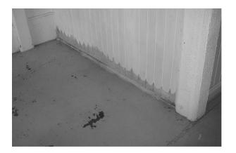
This wall was water damaged. An improvement in both waterproofing and surface drainage was required to rectify the problem.
