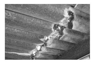
This rusting roof leaks every time it rains. A new roof is required.
