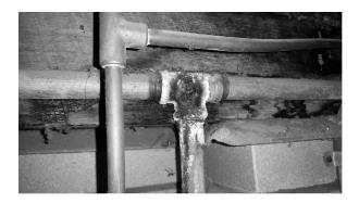
Rusting galvanised pipes are likely to also have rust in the inside. This can reduce water quality and pressure. Discuss the necessity of replacing galvanised pipes with your plumber.
