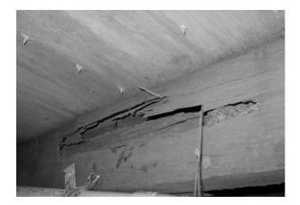
Subterranean termite damage to a hardwood floor joist. This joist had to be replaced.
