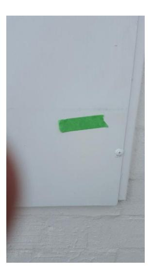
Seal gap to parapet flashing, right side, left of patio roof.
