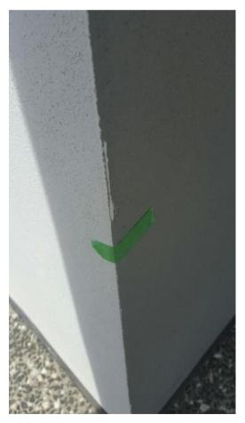
To Front Balcony, provide finish paint coat to timber beading, and repair damaged tile flashing.
