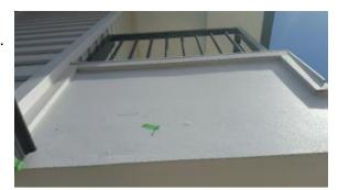
Repair gouges/lumps to left side of front balcony.
