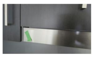
Seal gap above Refrigerator Recess cupboards and Pantry doors.
