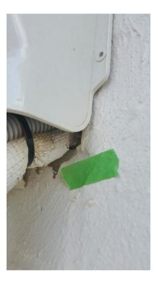
Remove plaster splatter to window / wall / downpipe, at left side.
