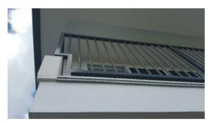
Front left, provide wider flashing (full width of gutter) above Garage door.
