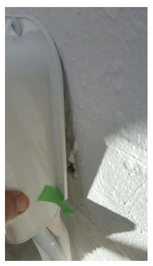
Touch up paintwork to higher aircon conduit penetration, left side.
