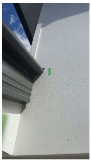
Repair paintwork and clean Downpipe, left side.
