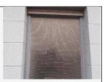
A section of louvres is missing to the rear elevation of the factory. Refer to sample photo. This is a Minor Defect. Repair or replacement is required. Consult a licensed tradesperson about the scope of works and cost to rectify.
