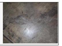
Concrete missing to top of blockwork under roller door openings. This could cause a person to trip. This condition has made this component a potential safety hazard. Suitable alterations should be carried out without delay to make this component safe.
