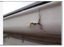
Gutters are damaged or rusting in sections. This will cause water leaks that can cause damage to other parts of the building. These should be repaired or replaced by a licensed Roofer or Plumber as necessary. Refer to sample photo.
