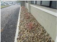
Drain cover missing to the Western elevation. This is a Minor Defect. Refer to sample photo. A licensed Plumber should further investigate this matter and provide a quotation for the necessary rectification.
