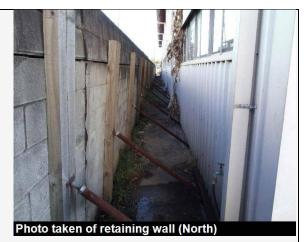
This wall does not appear to provide structural support to your building but does appear to support a section of driveway access to that Northern side of the building. For peace of mind I recommend that you have this matter further investigated by an appropriately qualified Structural Engineer prior to the contract becoming unconditional.
