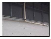
Gutters are damaged or rusting in sections. This will cause water leaks that can cause damage to other parts of the building. These should be repaired or replaced by a licensed Roofer or Plumber as necessary.
