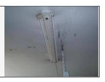
Some loose trims. This is a Minor Defect. Repair or replacement is required. Consult a licensed tradesperson about the scope of works and cost to rectify.
