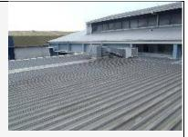
A small section of roof capping to the Northern end of the Office area roof is dented. Refer to sample photo. This is a Minor Defect. A licensed Roofer should further investigate this matter and provide a quotation for the necessary rectification.
