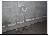
A steel roof beam has pulled away from the concrete block wall causing minor damage to the blockwall. Refer to sample photo. You should have this matter further investigated by an appropriately qualified Structural Engineer prior to the contract becoming unconditional.
