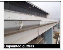
Paint has deteriorated on sections of downpipes and guttering. Repaint by a licensed Painter is recommended.
