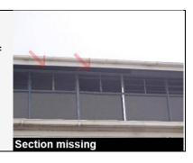
Concrete sun shade to front elevation is cracked in sections and this is allowing the penetration of some dampness. This is a Minor Defect. Repair or replacement is required. Consult a licensed tradesperson about the scope of works and cost to rectify. Refer to sample photo.
