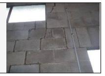
There are cracks in the blockwork. Refer to External Wall notes. Refer to sample photo.
