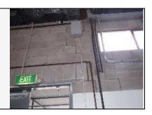
There is efflorescence (salt crystals) to the surface of the block wall. These crystals are the residue of excess moisture. This is a non-structural defect but dampness could be a problem. Further investigation by a Damp Control expert is recommended if dampness is a problem.
